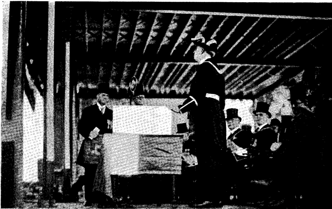
Corner-stone Laying of the Masonic Temple at Lowell, Massachusetts, September 8, 1928.
