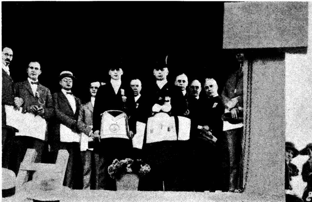
Laying the Corner Stone of Deaconess Hospital at Billings, Montana, August 15, 1923.
